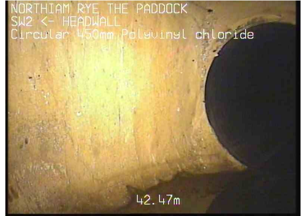
SW2_U_220225_095819__2.jpg, 00:06:21, 42.47 m Finish node type, manhole, reference number: SW2
