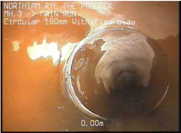
MH.3_D_220225_122742__33.jpg, 00:00:00, 0.00 m Start node type, manhole, reference number: MH.3
