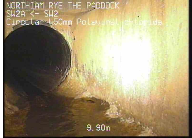
SW2A_U_220225_103517__4.jpg, 00:01:03, 9.92 m Finish node type, manhole, reference number: SW2A
